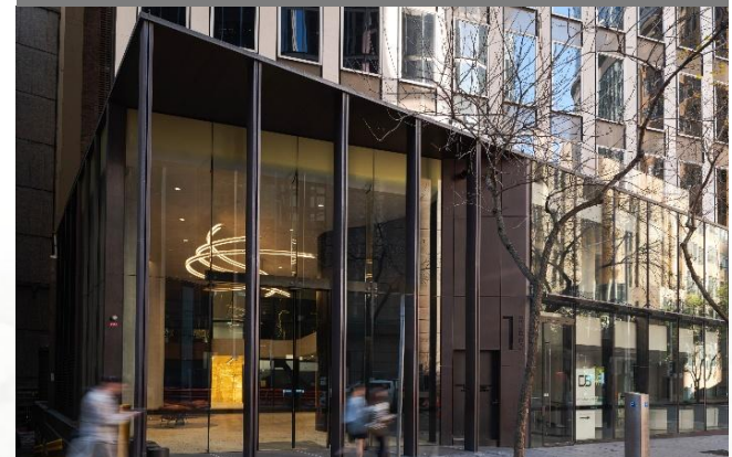
1 Castlereagh Street, NSW, Australia
