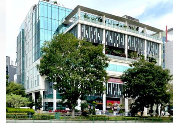
J’Forte Building, Singapore
